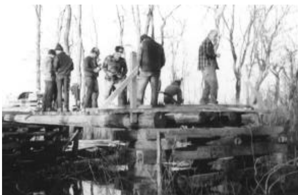
Building the Bark River Bridge in 1984
