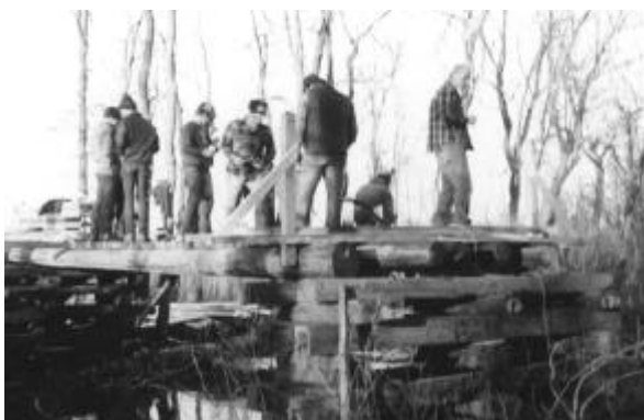
Building the Bark River Bridge in 1984
