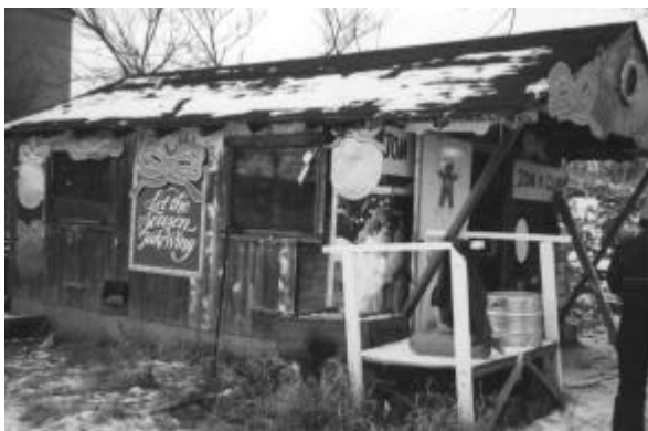
Trapp Farm Storage Shed
